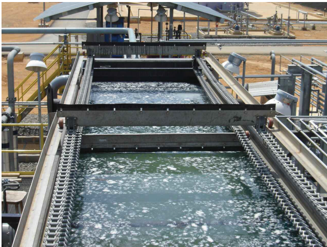
DAF with mechanical sludge scraper
