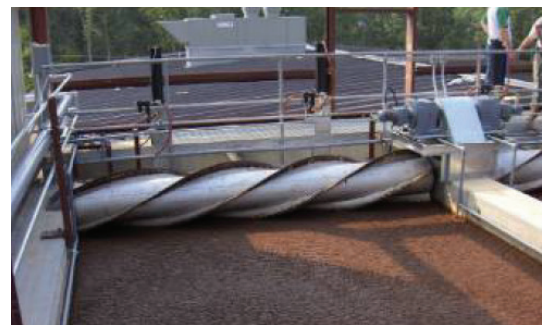
DAFF with hydraulic sludge decanting
